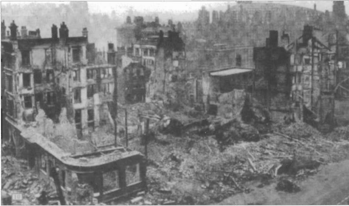
Damage to the Canon Street area.
