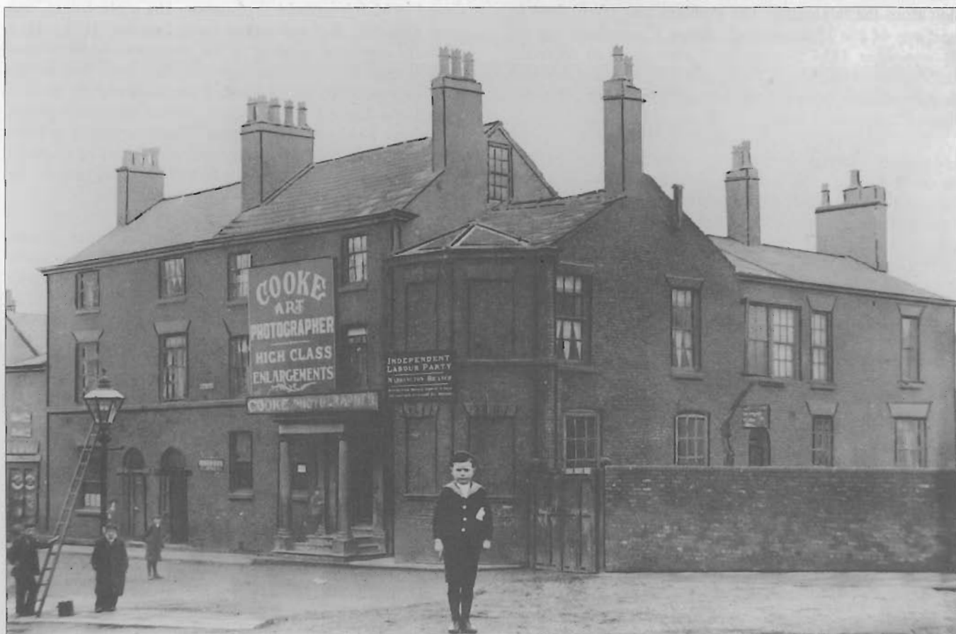
Later photograph of the premises in Friars Gate rented for the new Museum and Library 1848.
