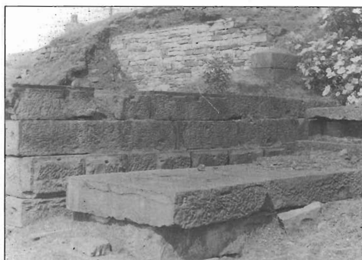
Brick pit shafts and engine bed, Tunsgill Colliery, Milnrow.
