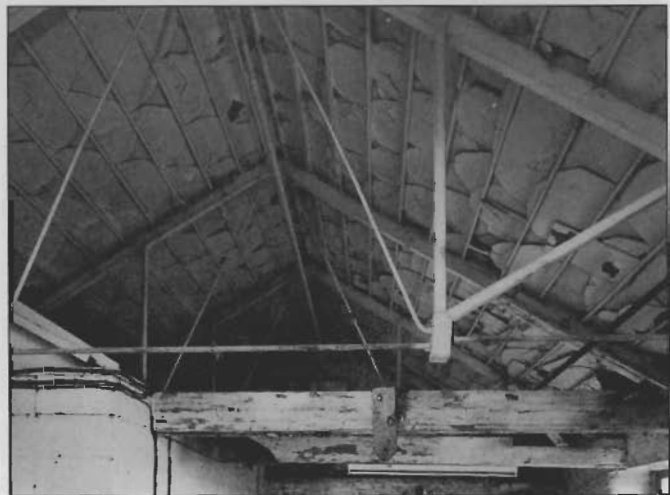
Combined cast-iron and wrought-iron truss construction in Beehive Mill's 1824 warehouse.
