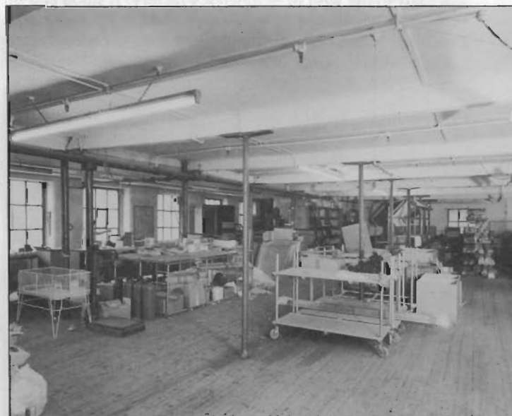
The interior of the Murray Street warehouse, complete by 1806, showing the original cruciform cast-iron columns.
