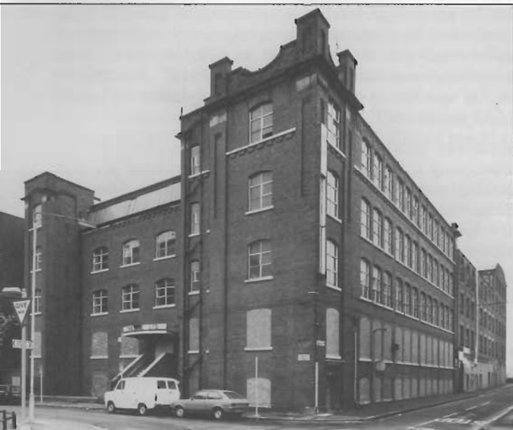
New Little Mill, added to Murray's site in 1908 for electrically-powered mule spinning.
