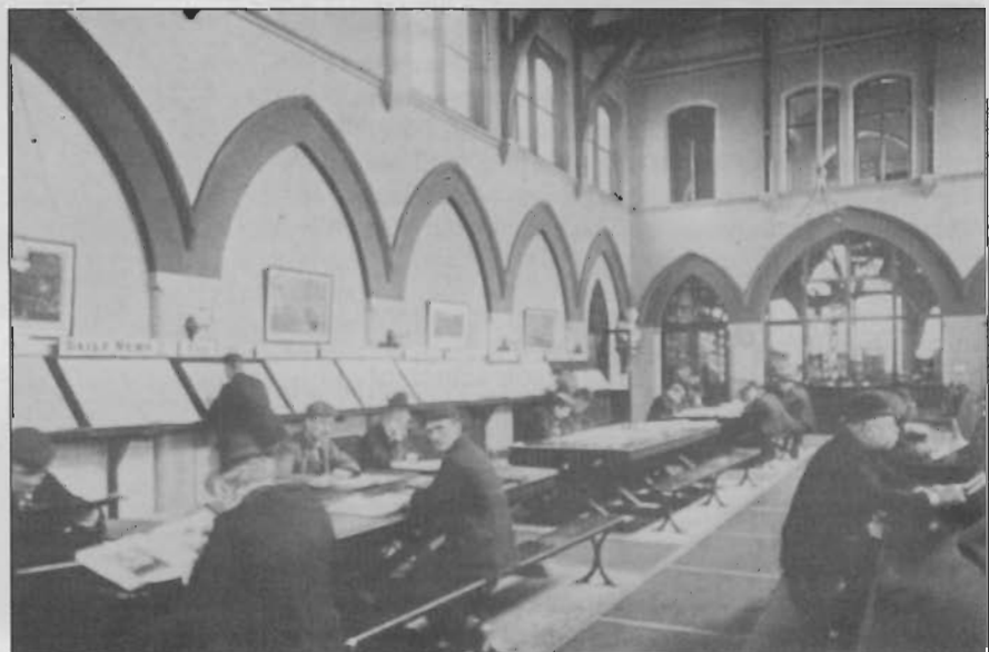
Ancoats Branch Library, Reading Room.
