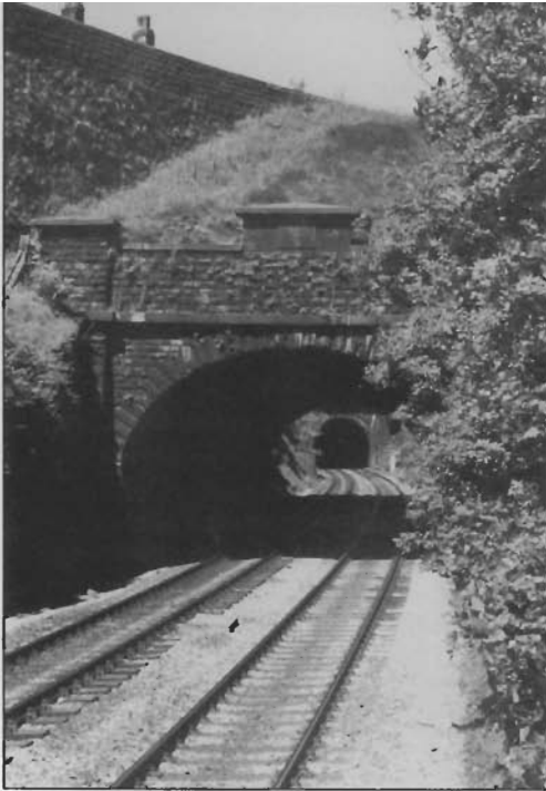
Summit Tunnel (W). The portal carries the only known example of the Manchester and Leeds Railway. Main Summit Tunnel beyond, opened 1841.
