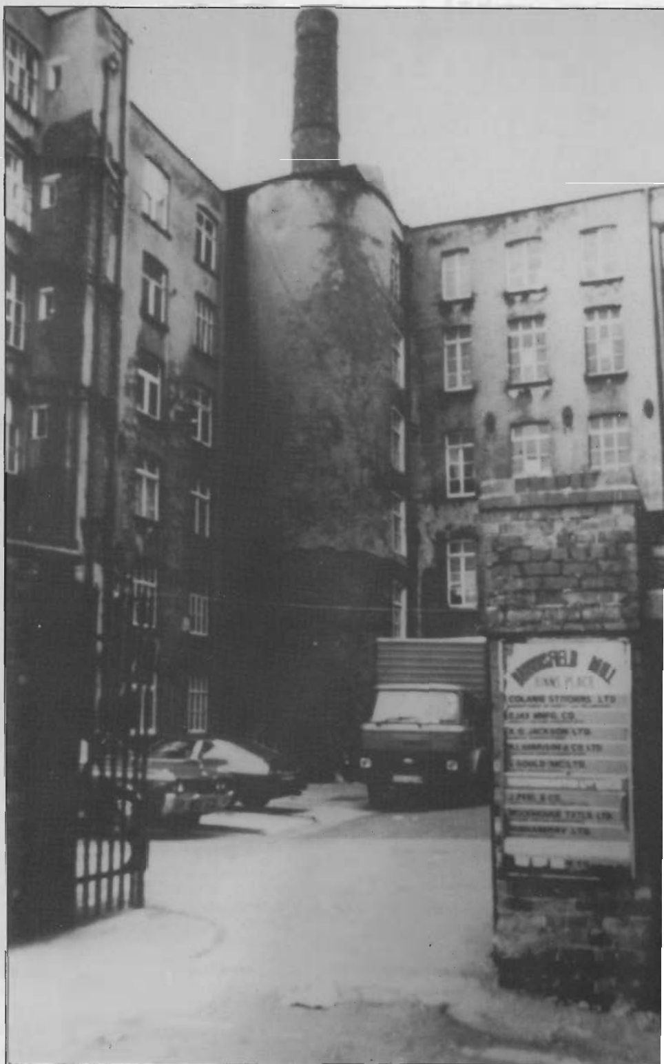
Brownsfield Mill, entrance to yard, showing stairtower.
