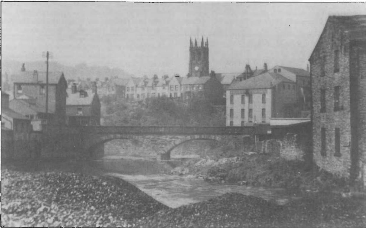
Station Road Bridge, Bridge End Mill (right).
