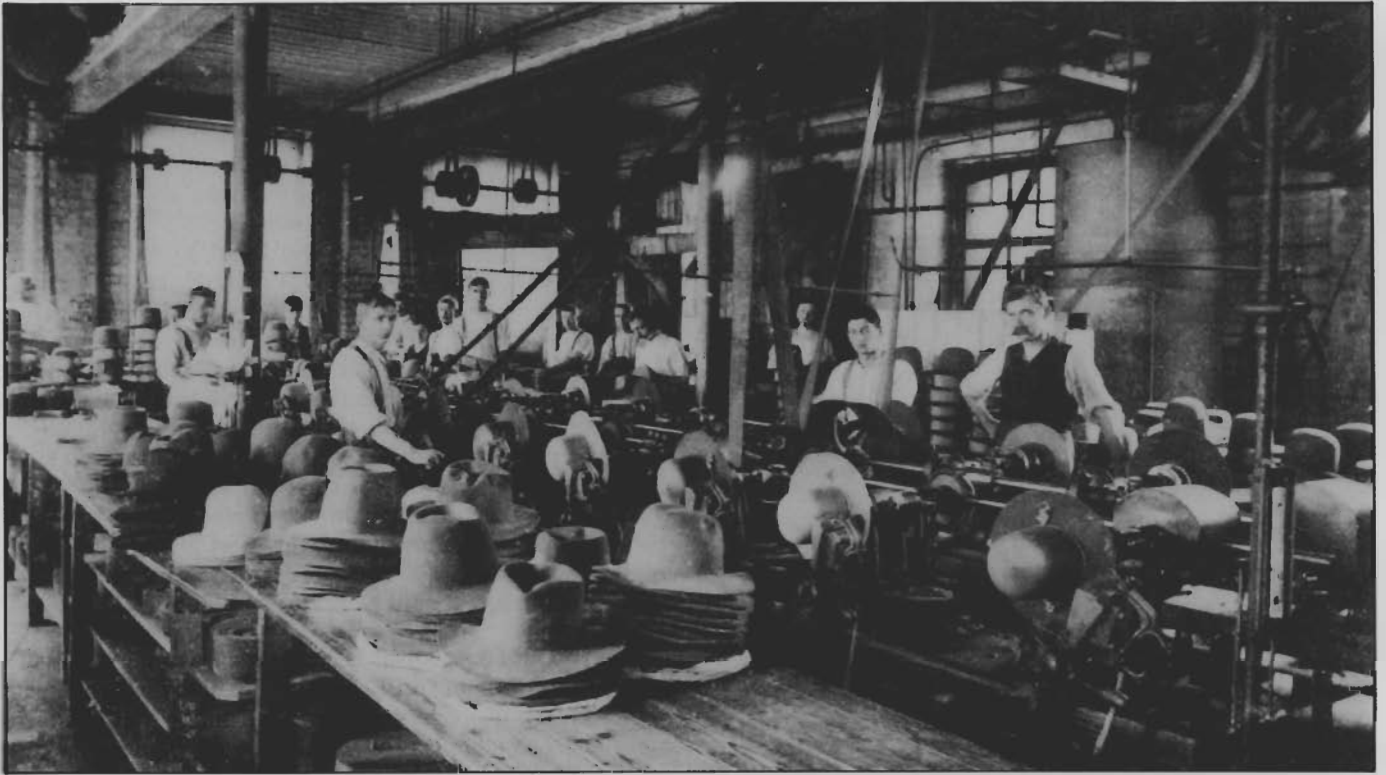
Battersby's hat factory, Stockport, 1911. The soft hat finishing room, where hats are smoothed by machine.
