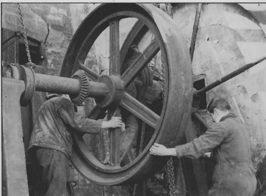
Removing the crankshaft of an 1860 'A-frame' vertical engine, Redferns Glassworks, Barnsley
