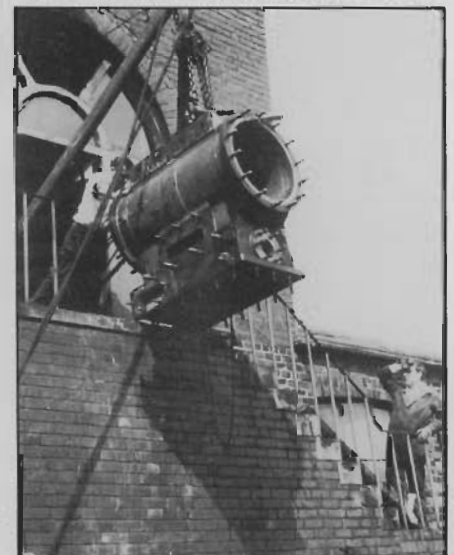
Cylinder of 1902 engine being removed from Wasp Mill, Wardle
