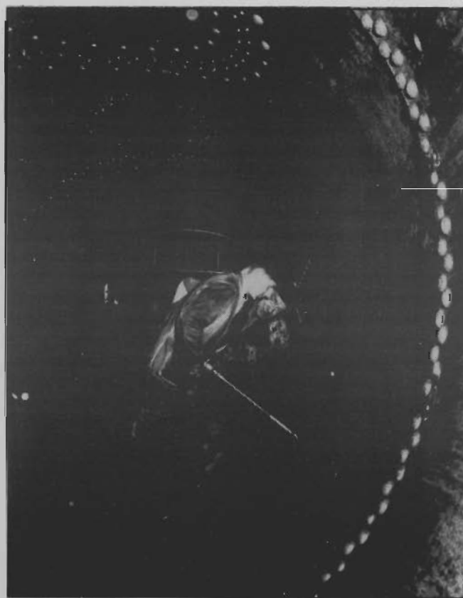
Riveting a boiler (Beyer, Peacock Collection)
