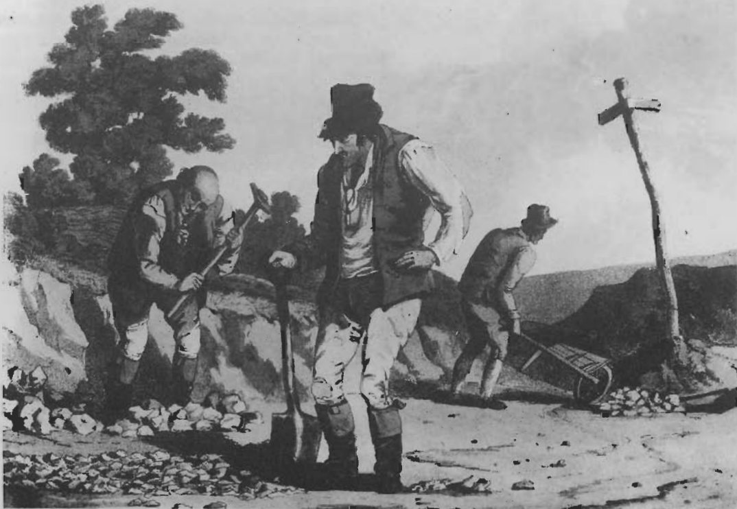
Stone-breakers at work on the road. An engraving from G. Walker, Costume of Yorkshire, 1814.
