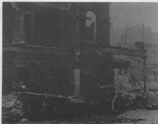
Leyland-Metz Turntable Ladder, damaged following a 'direct hit' on the building it was attending, Manchester Blitz, Dec. 1940.
