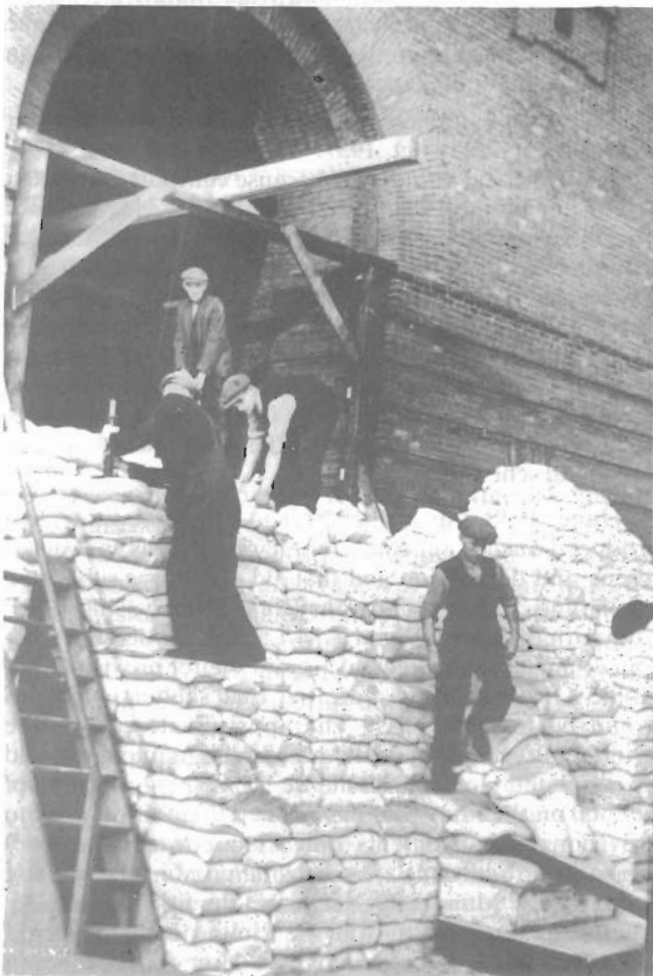
Sandbagging the railway arches.
