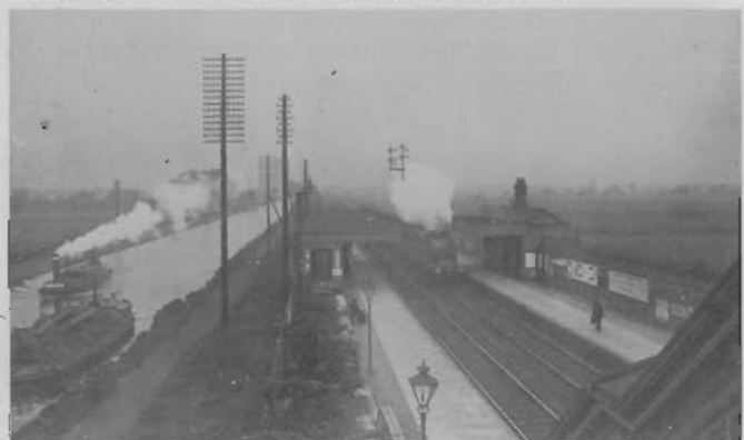
Timperley Railway Station.
