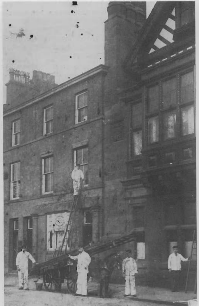
Altrincham and Sale Public Window Cleaning Company.
