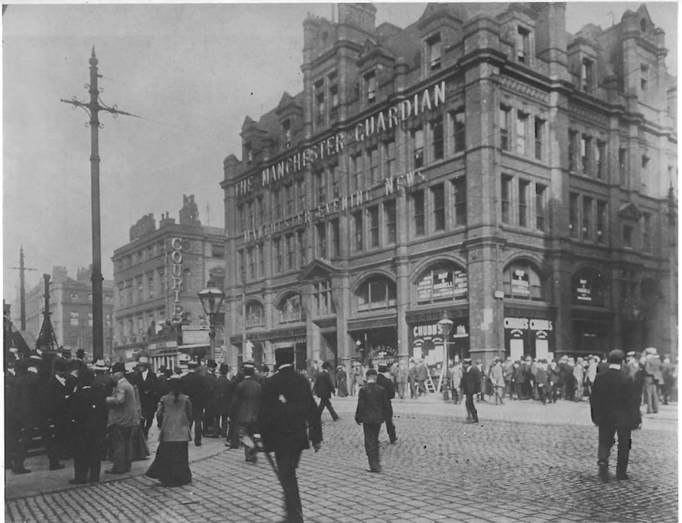
Although the offices of the Manchester Courier were on Cannon St., rivalry with the Manchester Guardian was such that the newspaper felt the need to buy advertising space on the building adjacent to the Guardian offices on Cross St., opposite the Royal Exchange building. Photo dates from 1902.
